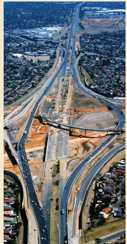
A work in progress...the EastLink - Monash Freeway interchange.
