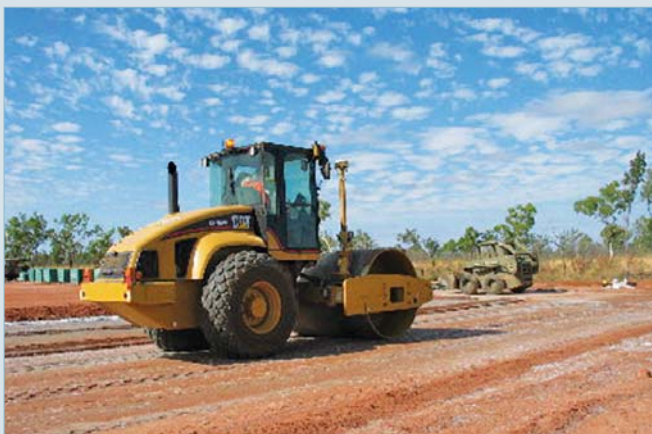
Cat Vibratory Soil Compactor mounted with AccuGrade technology.
