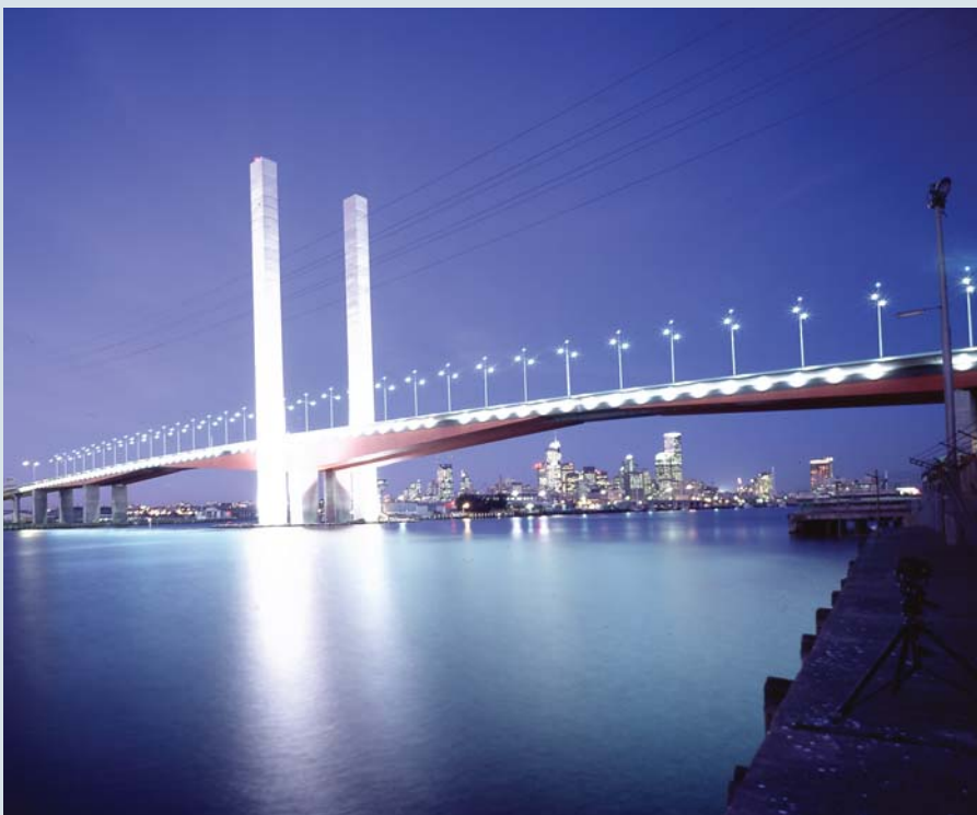
The Bolte Bridge, CityLink.
