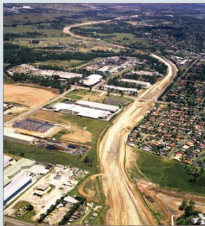
Construction under way on Westlink M7.
