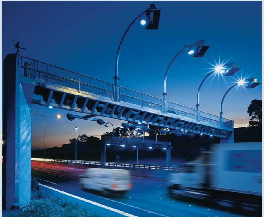
A fully electronic tolling gantry.
